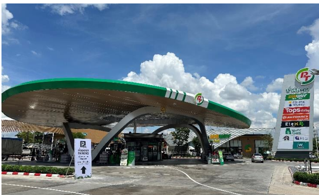
Exhibit 15: PT Max Rest station in Nakorn Pathom under Atlas
